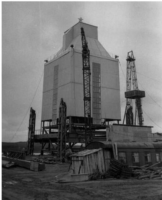
**Рис. 3. The tower gradually rises up with the help of four jacks (Kirshinbaum lift), new sections are added from below**
